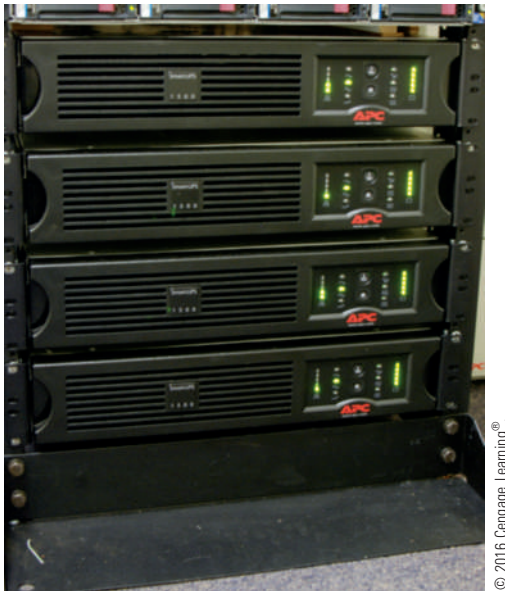
Figure 4-21 Online UPSs installed on a rack
