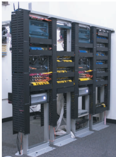
Figure 4-13 Two-post and four-post racks
