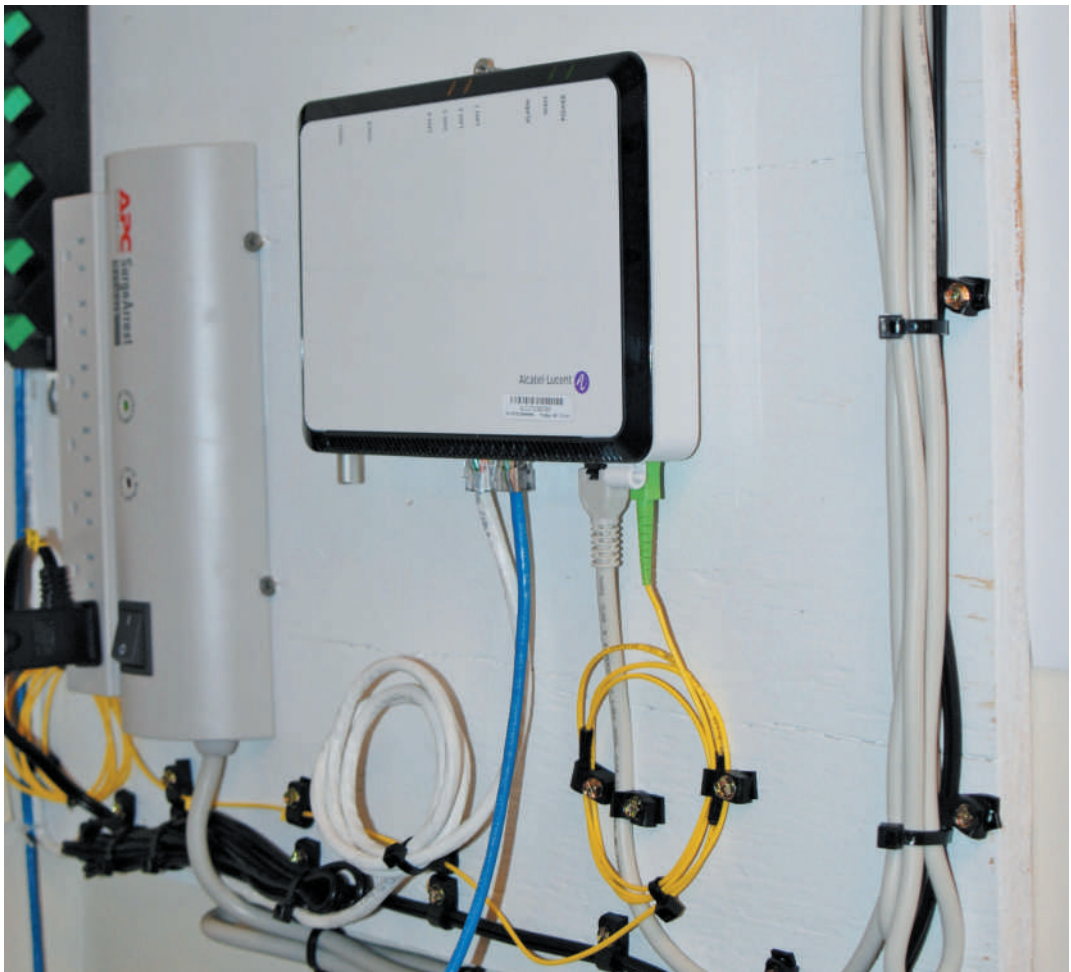
Figure 4-1 Demarc for Internet service to a campus network
